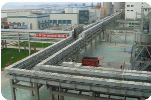
The application of non-segregated bus duct in power station
