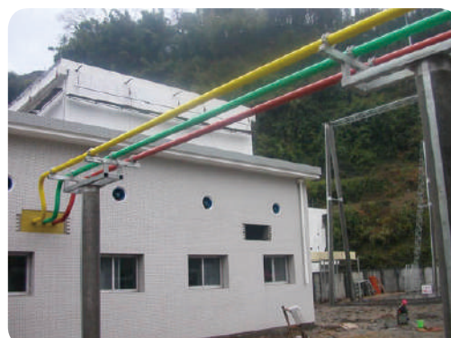
Application example 2 of the insulated tubular busway in the transformer substation
