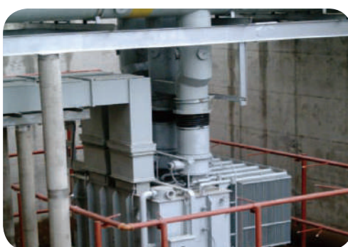
Auxiliary transformer connection
