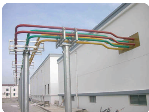
Application example 1 of the insulated tubular busway in the transformer substation
