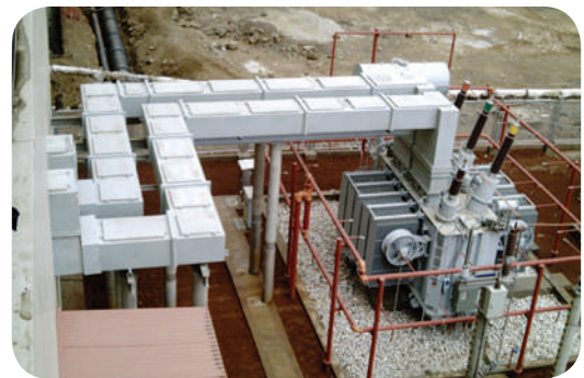
The application of non-segregated bus in start up and standby circuit
