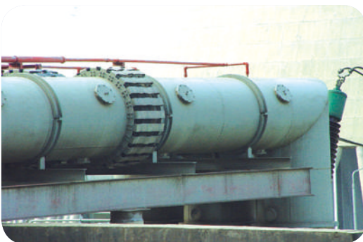
Removable expansion joint structure
