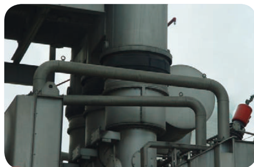
Main transformer connection
