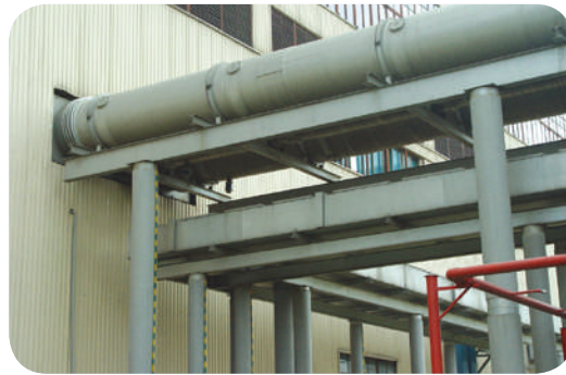
Wall-through seal and expansion joint structure
