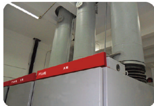
PT-LA cabinet connection
