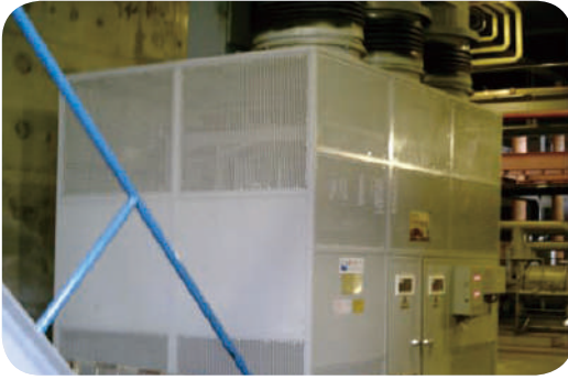
Excitation transformer connection
